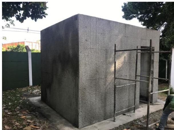
**Figura 22 – Parede chapiscada**
